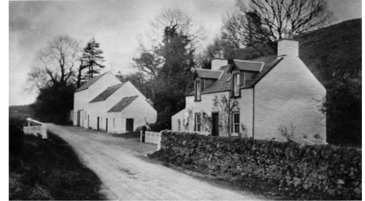
Barlay Mill & Miln of Barlay, Laurieston Road, Gatehouse
