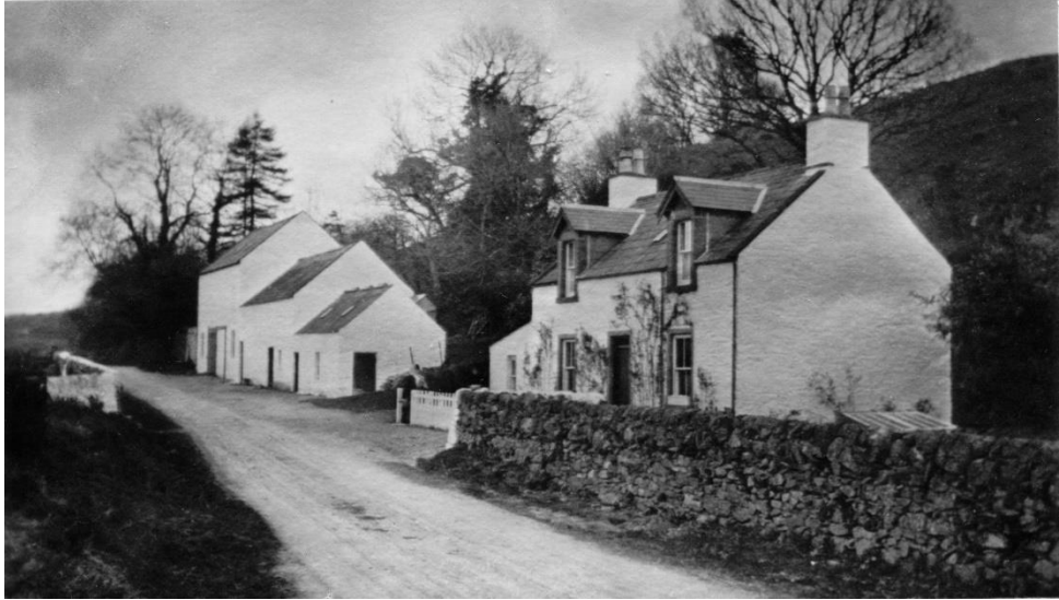
Barlay Mill & Miln of Barlay, Laurieston Road, Gatehouse
