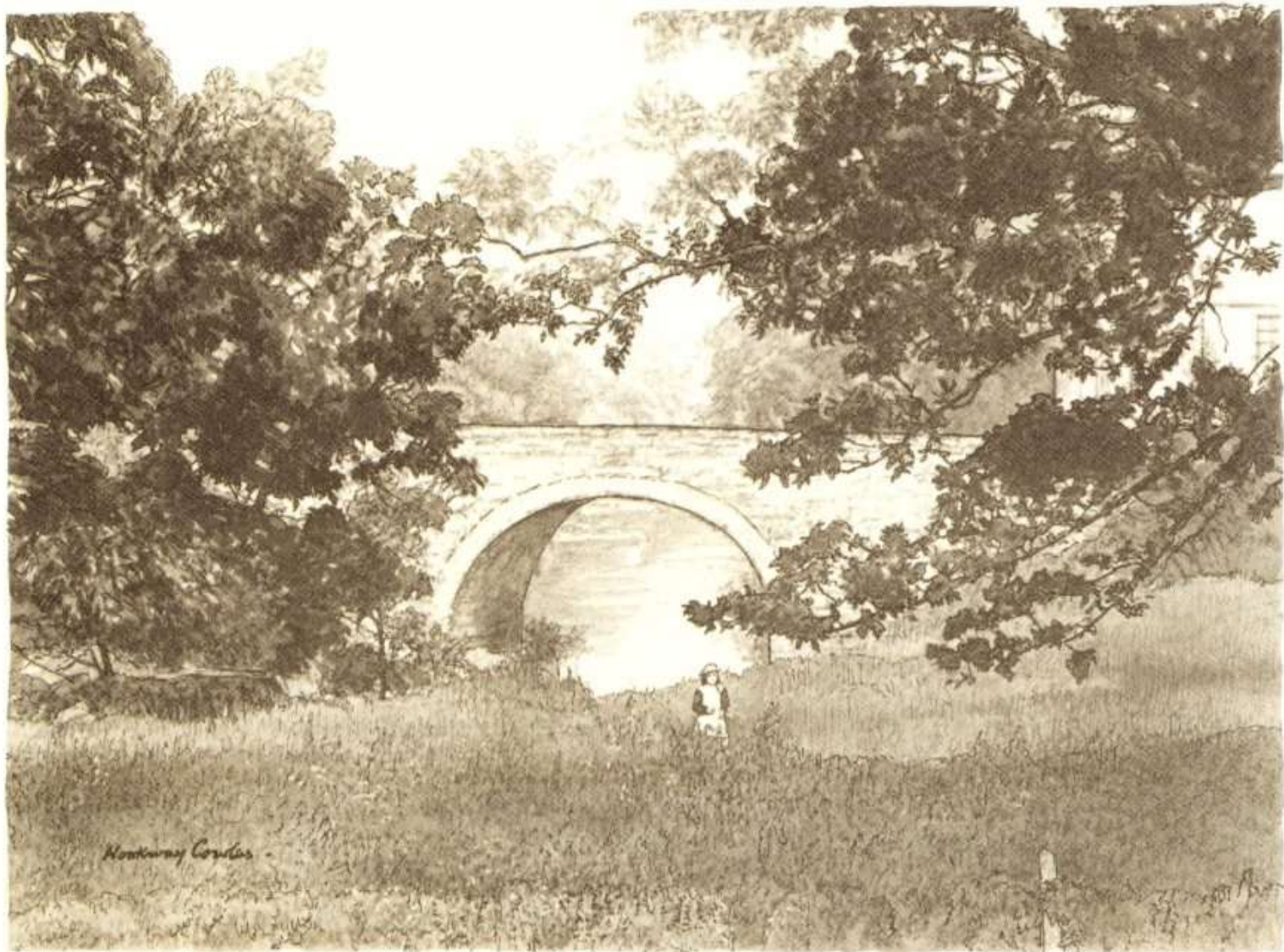
Old Fleet Bridge
